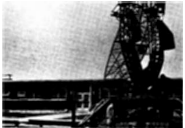
Figure 4. Height finder radar located near ground level.
